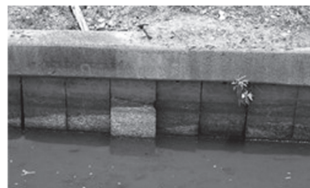
矢板ズレ傾き状況
